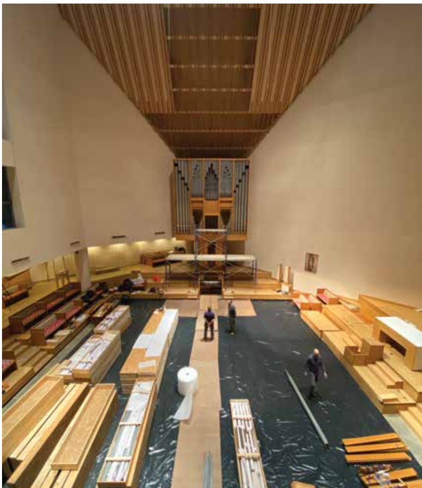
Pipework packing by the Organ Clearing House, with fine silt visible on floor beyond edges of plastic covering (photo credit: Jared R. Stahler)
